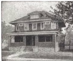
A No. 5-25-S IDEAL Boiler and 400 sq. ft. of 38 in. AMERICAN Radiators, costing owner $220, were used to heat this cottage. At this price the goods can be bought of any reputable, competent Fitter. This did not include cost of labor, pipe, valves, freight, etc., which vary according to climatic and other conditions.
